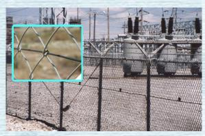
The PIDS provide surveillance of industrial or governmental site perimeter wall/fence including all entrance gates and exits. The offered IDS will be able to function as a standalone system or as an integral component of a centralized security system. The system operates normally during the day and night, in all weather conditions, including sand storms.
