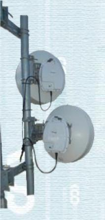
A microwave link is a communications system that uses a beam of radio waves in the microwave frequency range to transmit information between two fixed locations on the earth, distance between the microwave stations can be from just a few feet or meters to several miles or kilometers apart. Also a Microwave network can be in the form of Point to Multipoint communication is often abbreviated as P2MP, PTMP, or PMP.
